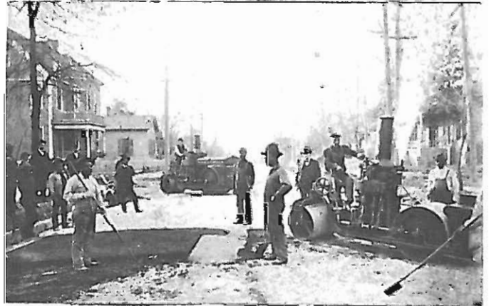
Street paving projects in the early years always attracted a large crowd of on-lookers.
