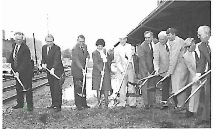
Officials shovel gravel to officially begin work on the Pine Bluff railroad relocation project.
