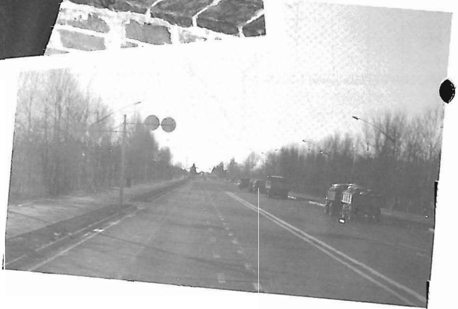
A "typical" Chinese highway north of Beijing. Separate bicycle roadways are constructed along the outside of the traffic lanes.
