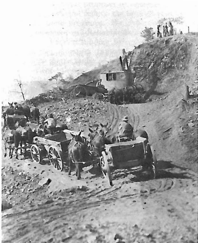
Early construction work on the State Highway System required lots of man- and horsepower.
